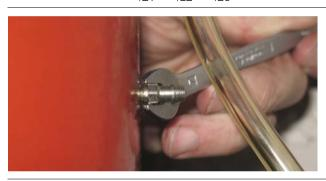
9. Tighten the air-bleed screw when no more air is escaping
