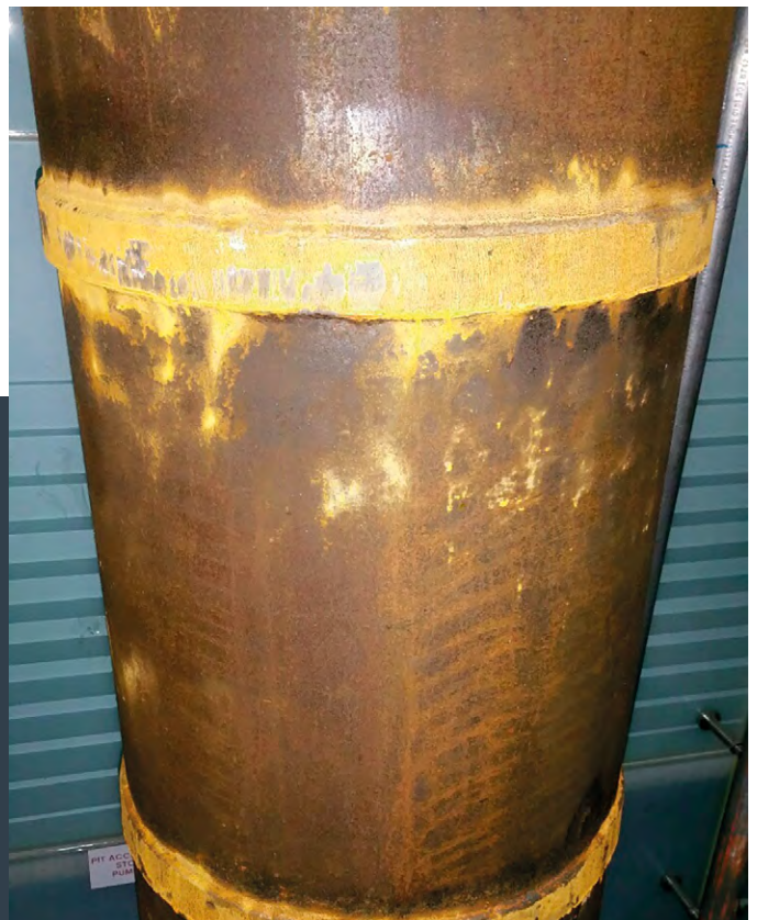
top image Steel sleeve pressed into place, liner being readied for lowering into sleeve · bottom image Steel liner welded and ready for lowering into the sleeve
