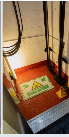
After receiving instructions from the lift service provider, we decommissioned and removed the existing lift and its ancillary equipment. Our installation team cleaned and redecorated the lift shaft and drive/pump room, located in the buildings gated car park. We re placed all of the hydraulic equipment in the shaft including the ram and installed new shaft lighting. Also, we installed new landing entrances including builders work and car doors, new lift car and finishes, energy
